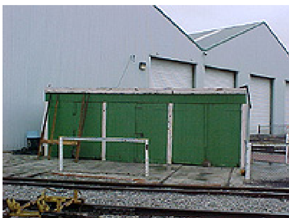
Eudunda gangers shed
